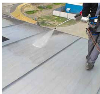
Preparation of the surface with high pressure water
