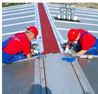
Sealing an industrial roof
